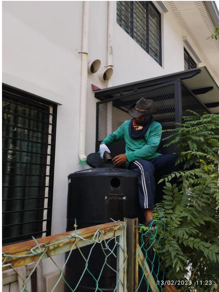
Rajah 25 professional memasang skrin mesh kalis nyamuk
