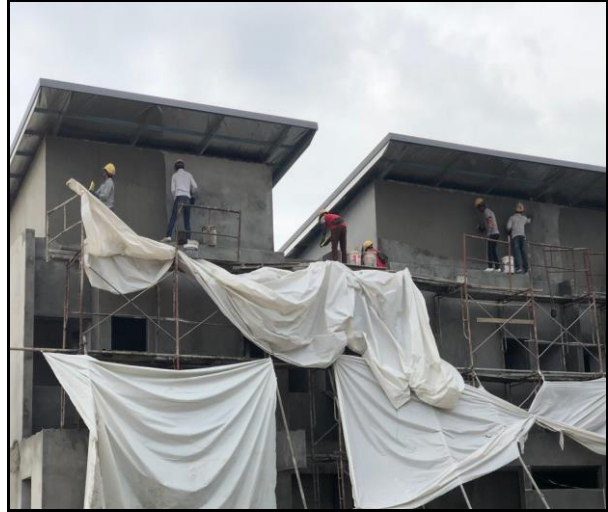
Picture 4 : Scheme Coating & Plastering Works (Outside)
