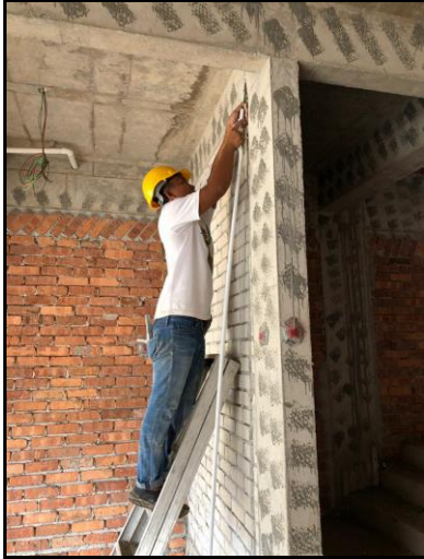
Picture 3 : Plastering Works
