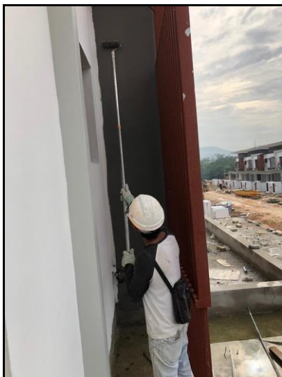
Picture 1 : Painting Works
