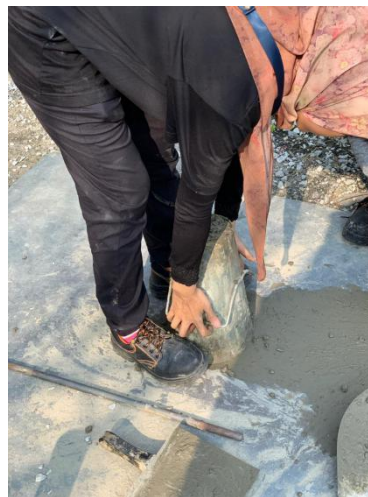
Figure 3.6 : The Cone is Pulled in Parallel
