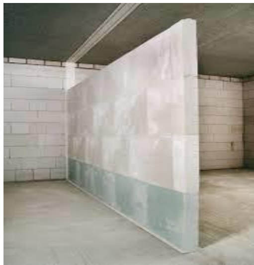
Figure 5.3 : Concrete Partition Wall
